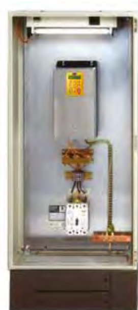
DC590+ DRV equivalent illustrating panel space saving
